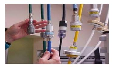
Unique connectors ensure medical gas hoses will be connected only to the appropriate gases.
